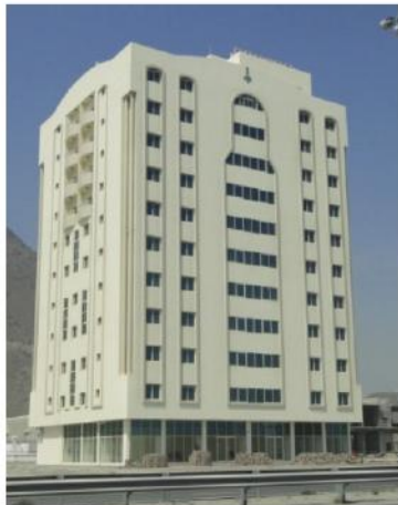
G+10 MULTI STOREY BLDG Contractor: ASIAN CONTRACTING
