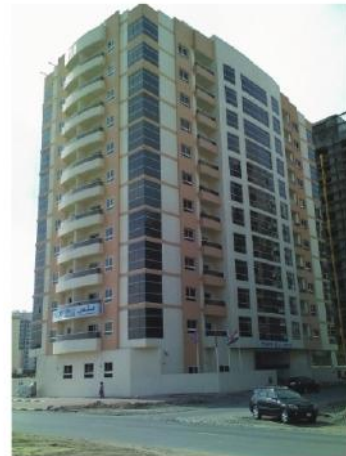
G+11 MULTI STOREY BLDG Contractor: BIN ZAYED CONT.
