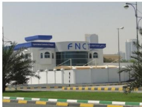
FNCT OFFICES Contractor: FNCT
