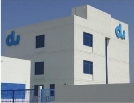
DU-FUJAIRAH CABLE LANDING STATION Contractor: AMANA STEEL
